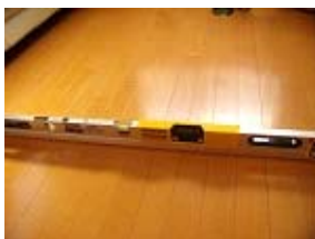
床の傾きを水準器で計測
